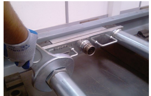
5. Securing the PTW into the track.
